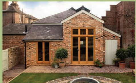
HISTORIC BUILDINGS RESTORATION . RENOVATION REPAIR
