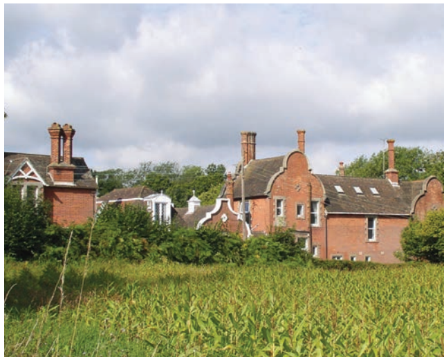
Back of the estate office, coach house and stables today
