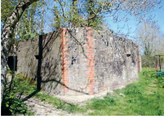
Pill box at Lindfield Bridge
