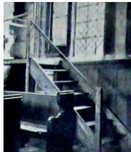
Emergency exit in All Saints church
