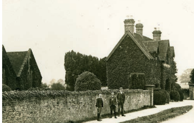
View of Entry Lodge c1900
