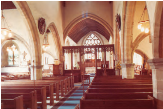
Nave with Chancel Screen in Chancel Arch
