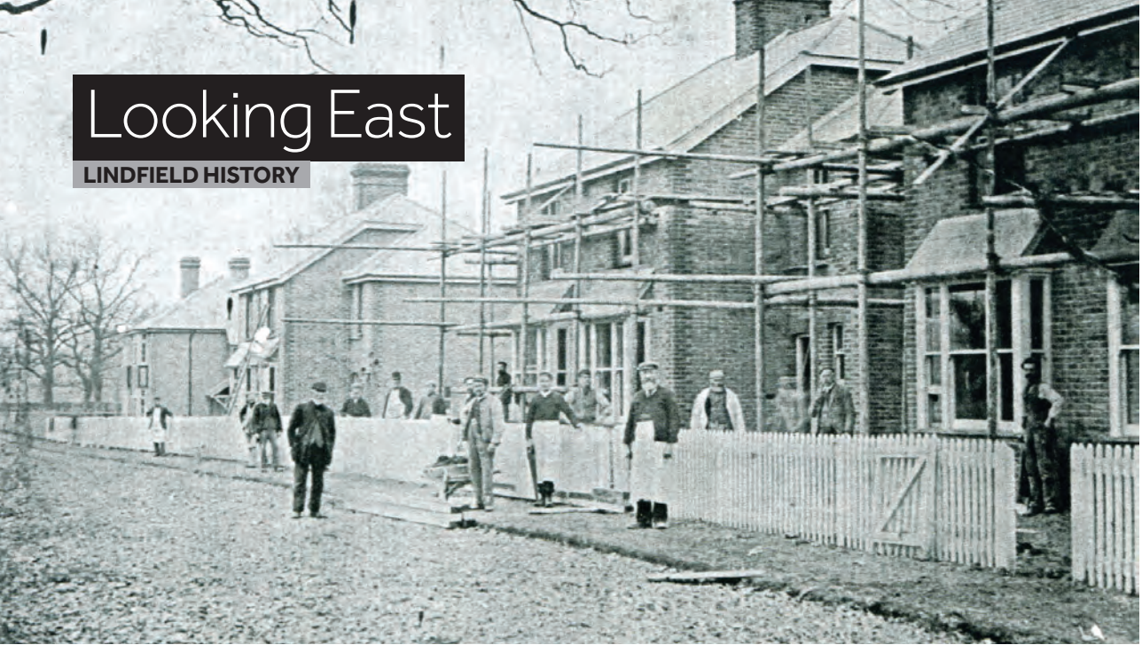
The first houses in Eastern Road under construction
