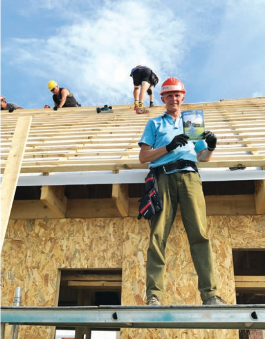
Chris Rigby Smith building a house in Oradea, Romania
